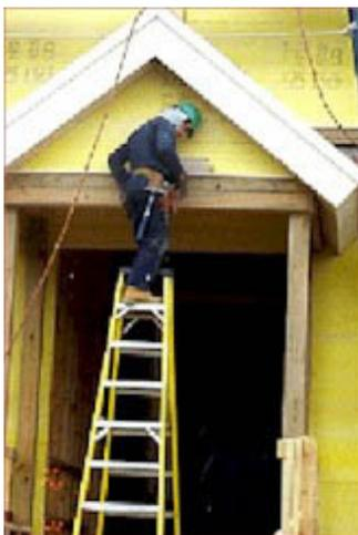
This is improperly using the top rung of this step ladder to work from.
